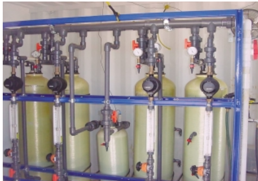
The AVRWC pilot arsenic removal plant is being used to demonstrate the capability of new technologies to effectively and economically remove arsenic from well water.
