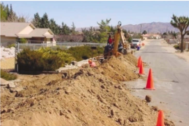
The job above involved replacing 480 feet of six-inch diameter water main, replaced on Haida Rd. While this job was an emergency replacement, AVRWC has a master plan to prioritize and schedule infrastructure replacement.
