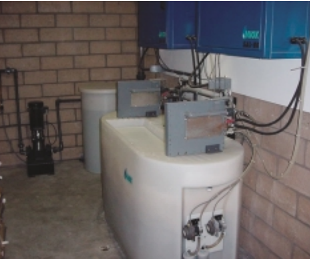
New MIOX disinfection technology is being installed at AVRWC wells. This advanced, mixed oxidant system makes low, non-hazardous concentrations of chlorine disinfectant from salt on-site. Superior disinfection is achieved with lower doses and with less taste and odor to the customer. This process also improves worker safety by eliminating the need to handle large quantities of liquid chlorine.
